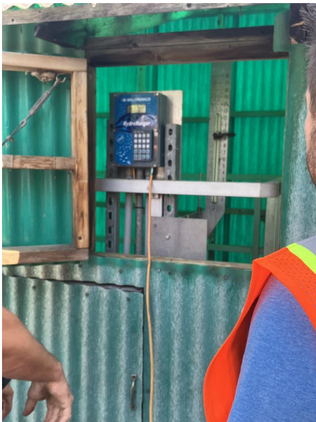
7- New Flow Meter with Temporary Wiring
