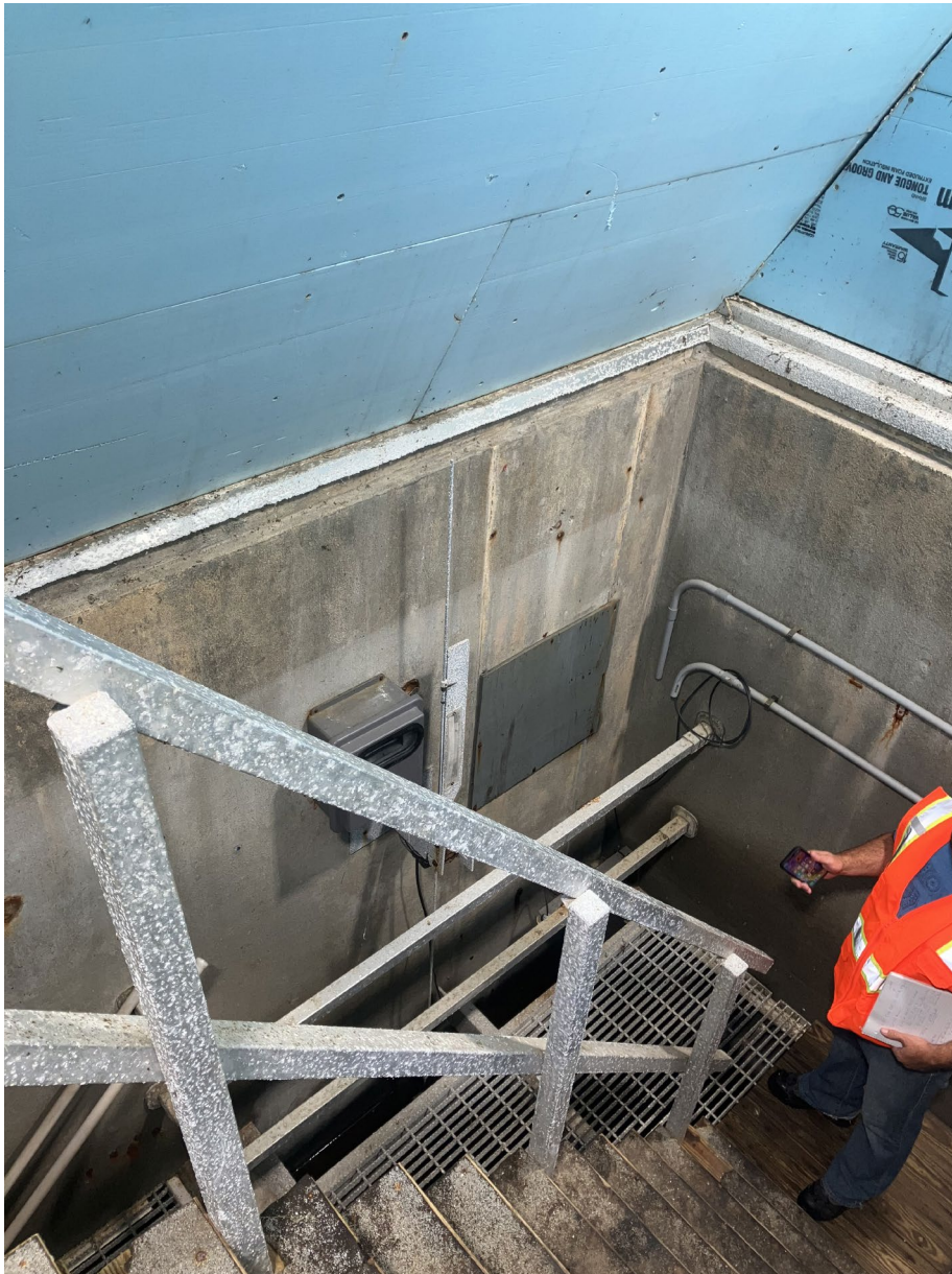
1- Old Flow Meter (Note Flood Water Line Was 12 Inches Above Meter as Depicted by the Lighter Gray Line on Wall)
