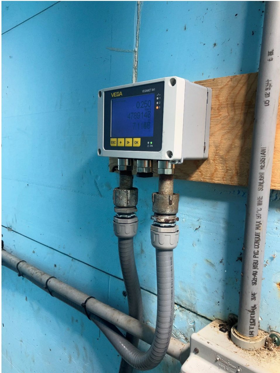
2- New Flow Meter Elevated to Above Grade Just Inside the Doorway of the Outfall Building
